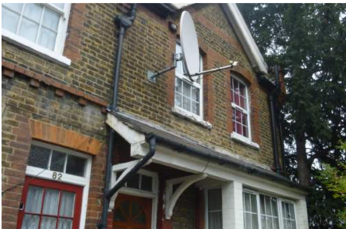
Satellite dish and replacement windows
